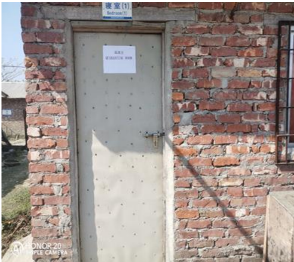
Figure 35: Quarantine room of Polder 43/2C
