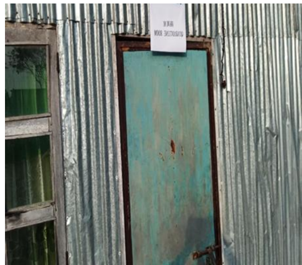
Figure 34: Quarantine room of Polder 41/1
