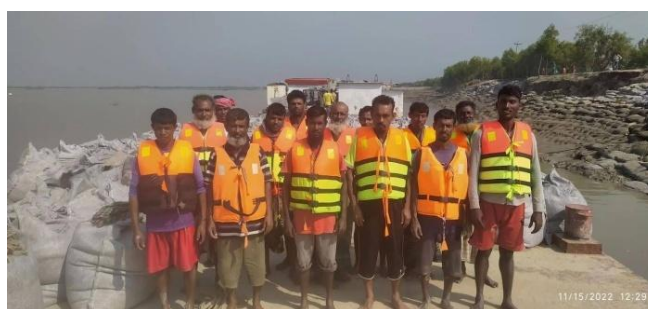
Figure 16: Safety arrangements for emergency works (P-32)
