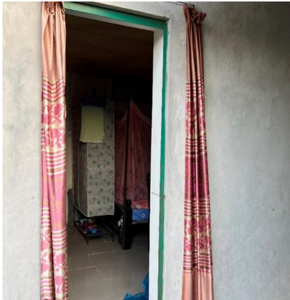
Figure 31: Quarantine room of Polder 39/2C
