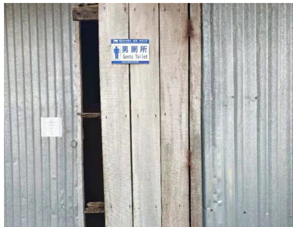
Figure 37: Toilet facility of Quarantine room of Polder 48
